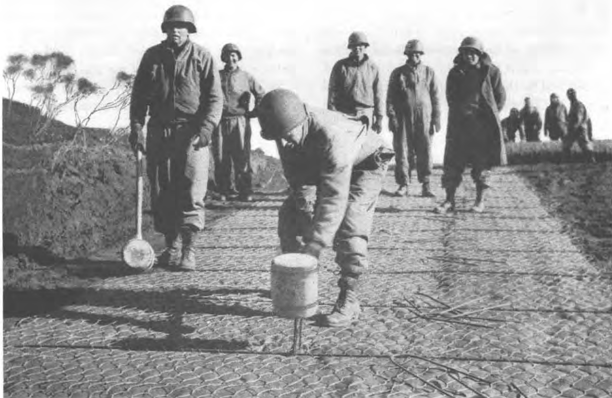
PUTTING DOWN ROAD MATTING at the beach exits was one of the problems confronting the engineers after the landings. Many heavy vehicles and the rapid supply build-up made the construction of a number of such roadways necessary.
