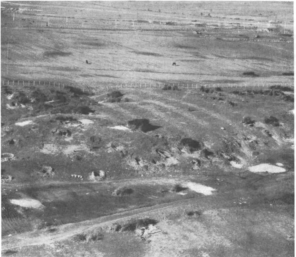
DUGOUTS ALONG THE MUSSOLINI CANAL had been fairly well prepared in every defilade. From positions such as these the 1st Special Service Force was able to stem enemy attempts to breach the right flank.
