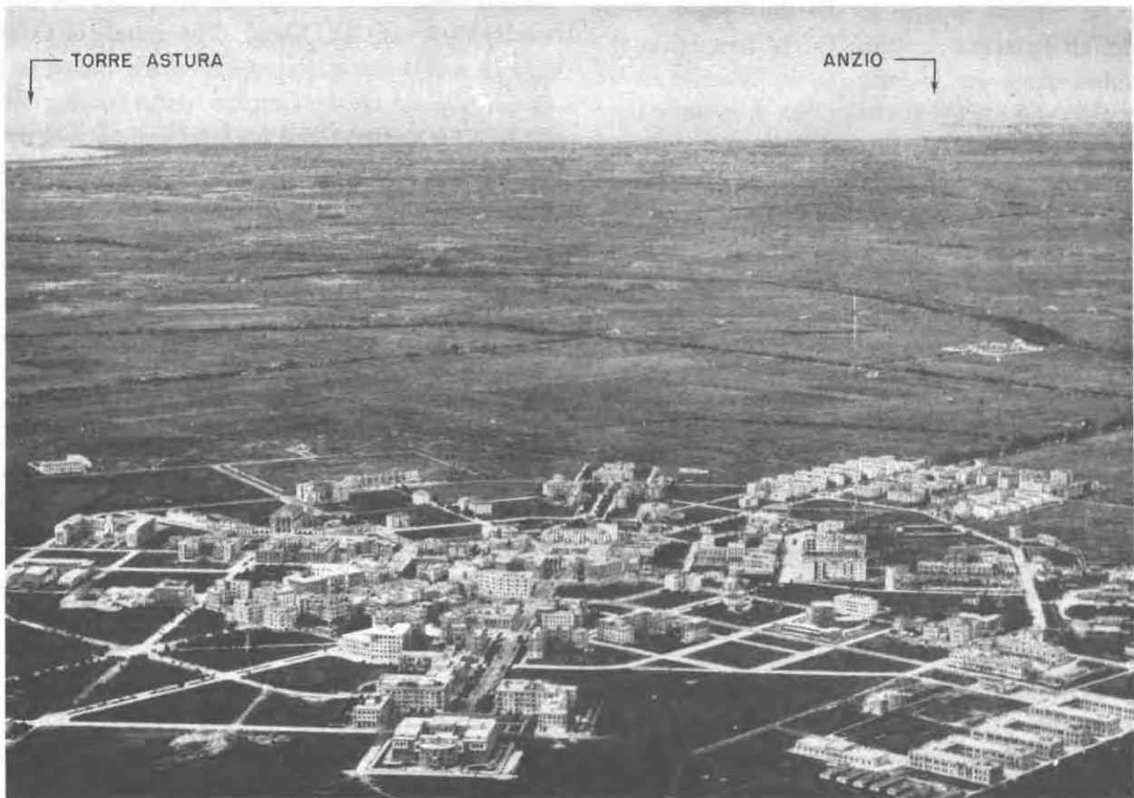
LITTORIA AND THE RIGHT FLANK of the beachhead, viewed from the air. The Mussolini Canal flows from right to left across the terrain shown in this photo, about one-third of the distance between Littoria and Anzio. The Factory (Aprilia) was very similar in structure, and built about the same time as Littoria.
